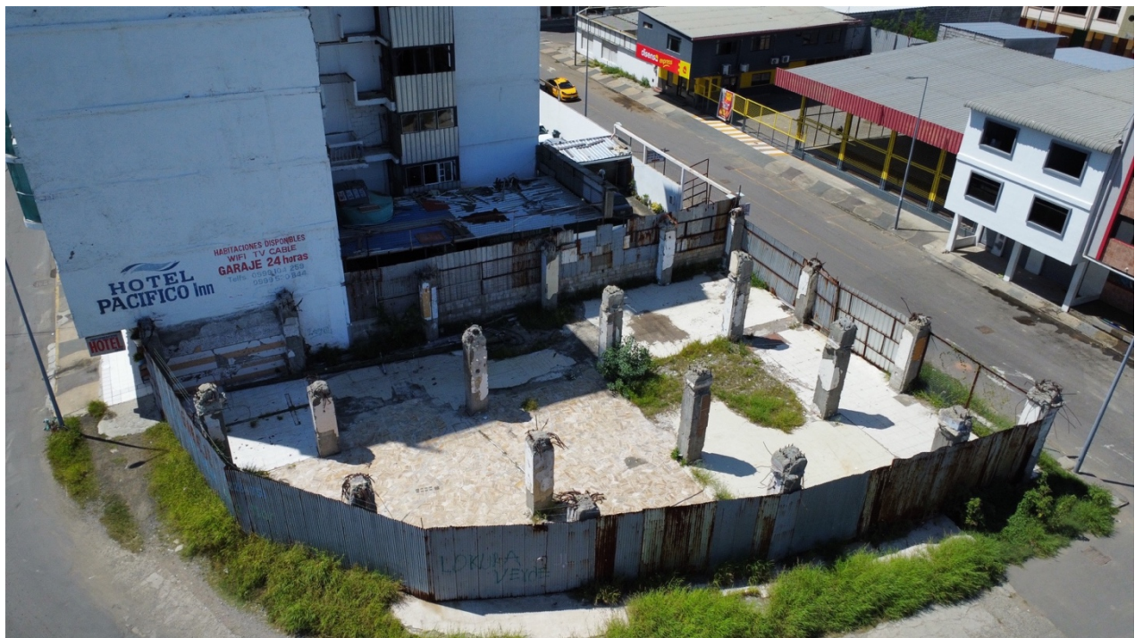
Fig. 10. Destroyed building due to 16A in Tarqui
