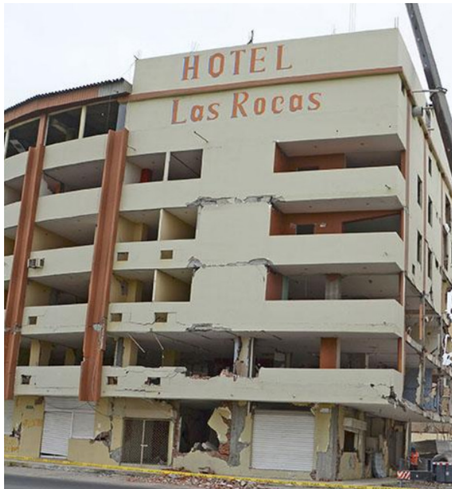
Fig. 8. This is how the building looked after the earthquake in Tarqui, due to the collapse of two floors it was decided to demolish it.
