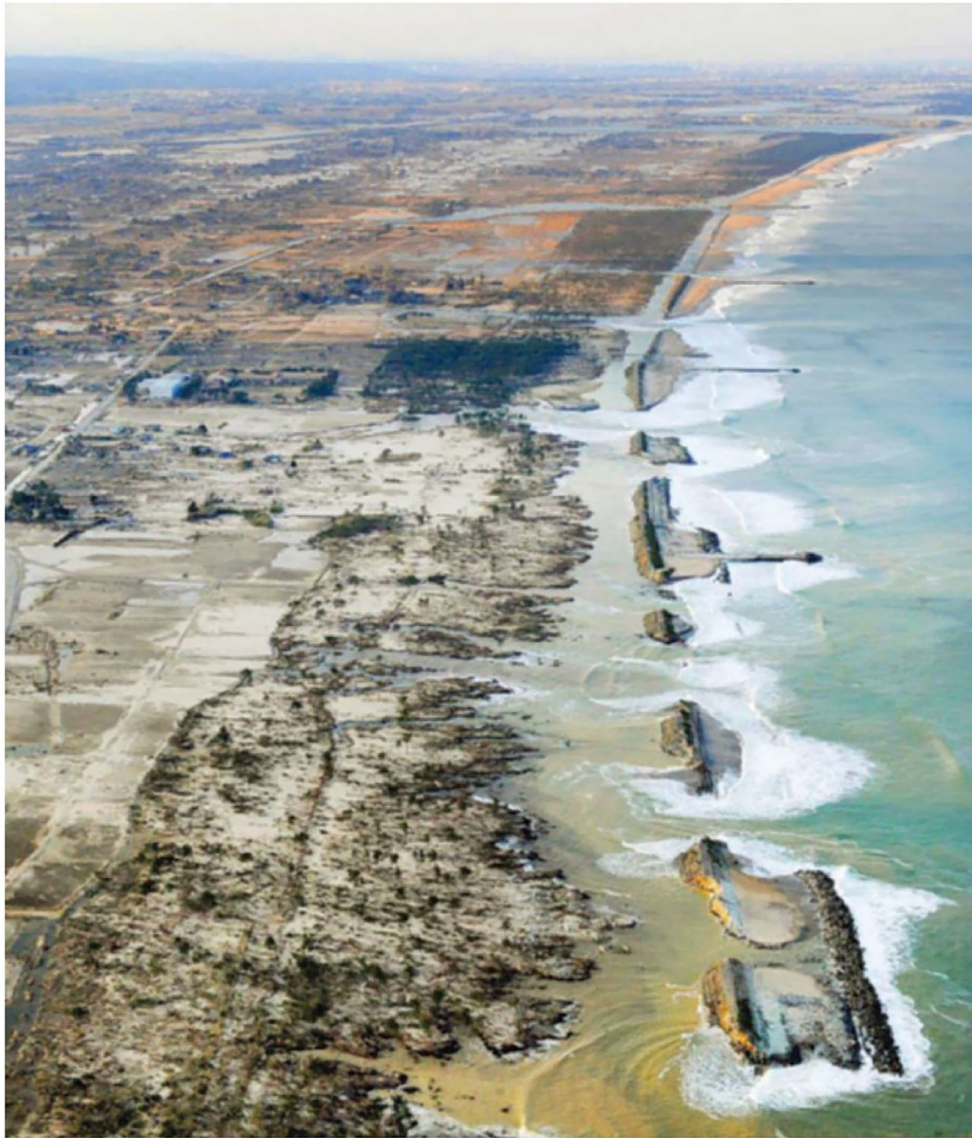
Fig. 1. Seawall destroyed by a tsunami (Mano et al. 2013)
