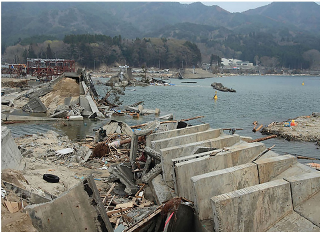
Fig. 2. Seawall of a harbor in Yamada completely destroyed by a tsunami.
