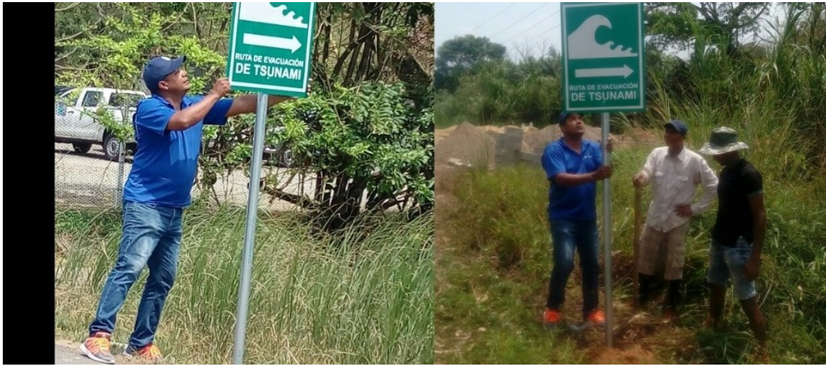
Fig. 6: Installation of Tsunami evacuation signs in Panama. Credit Critica.com.pa
