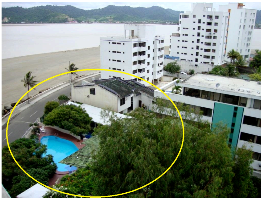
Figure 22: Homes located between buildings on the pier "Virgilio Ratti".
