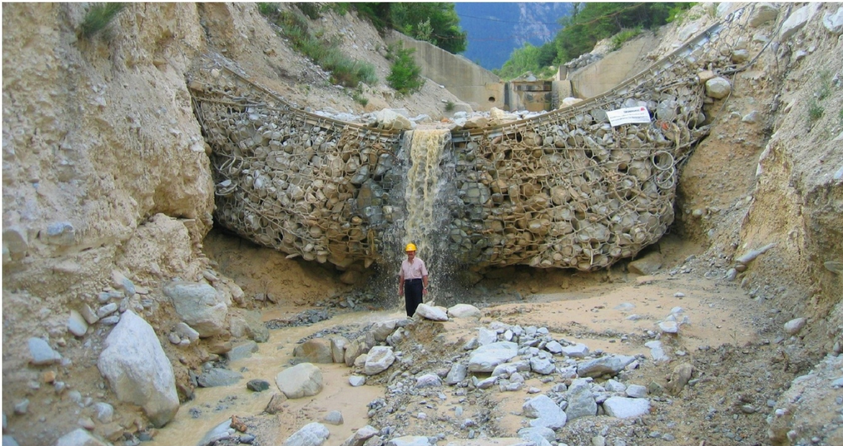
Figure 4. Landslip stopped by high-strength steel fence
