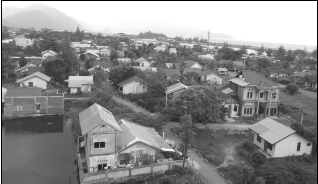
Figure 1. View of new buildings after reconstruction around the coastal area of Ulee Lheue Banda Aceh. The houses are recently built for tsunami victims (taken from newly built escape building on January 2013).
