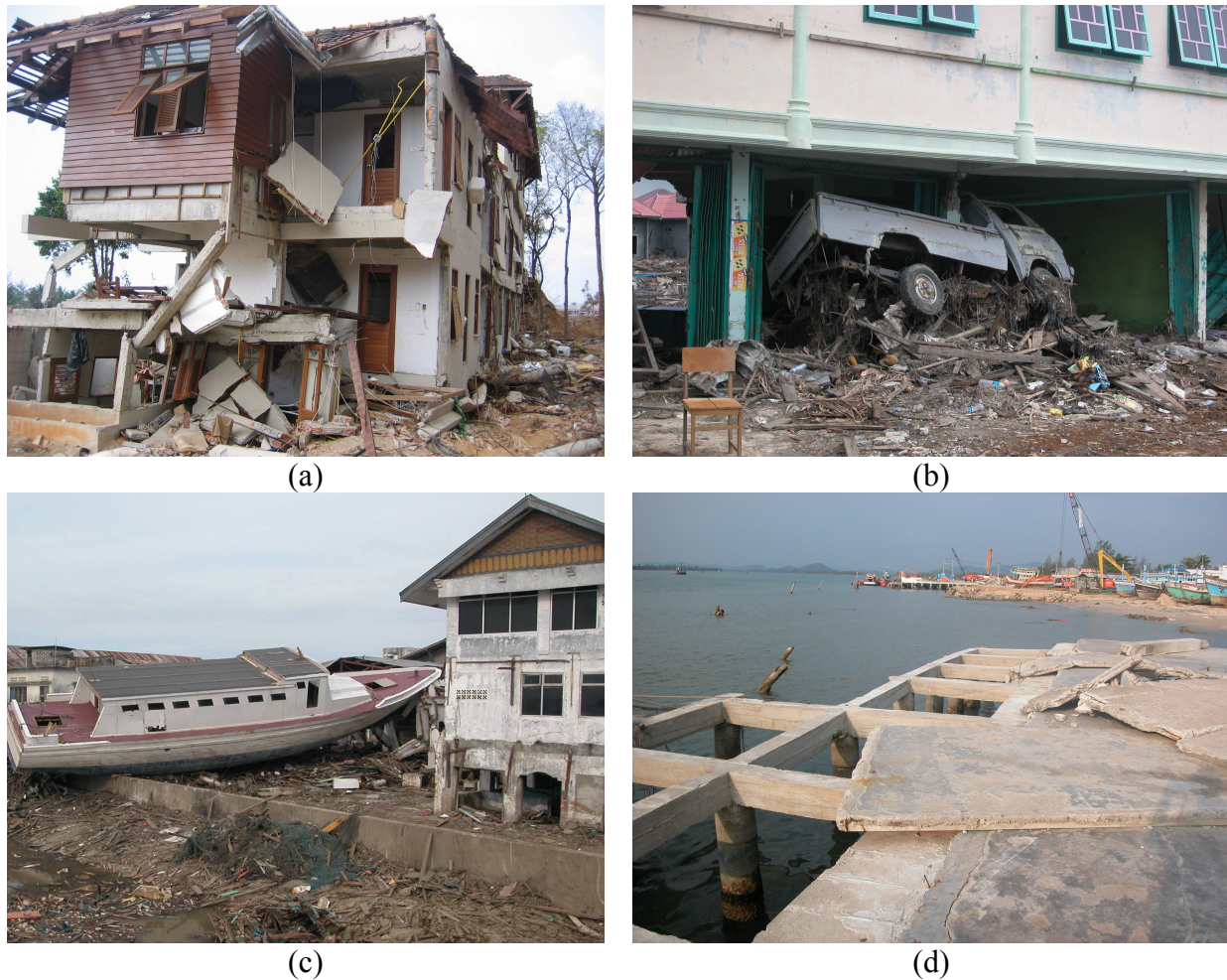
Figure 1. Effects of 2004 Indian Ocean tsunami on structures (Saatcioglu et al., 2006a, 2006b): a) global damage to non-engineered concrete residential structure in Phuket Island, Thailand; b) debris impact and damming in Banda Aceh, Indonesia; c) debris impact from large vessels in Banda Aceh, Indonesia; and d) uplift of concrete slabs in Khao Lak, Thailand.
