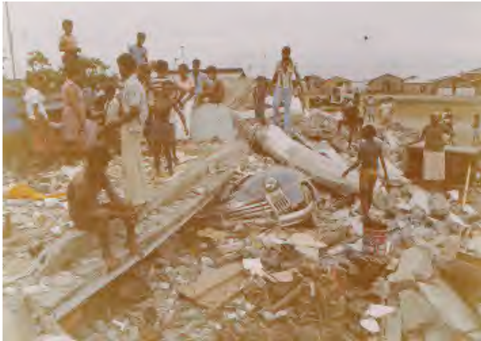
Figure 3. Earthquake damage at Tumaco, Colombia (photo by G. Pararas-Carayannis)
