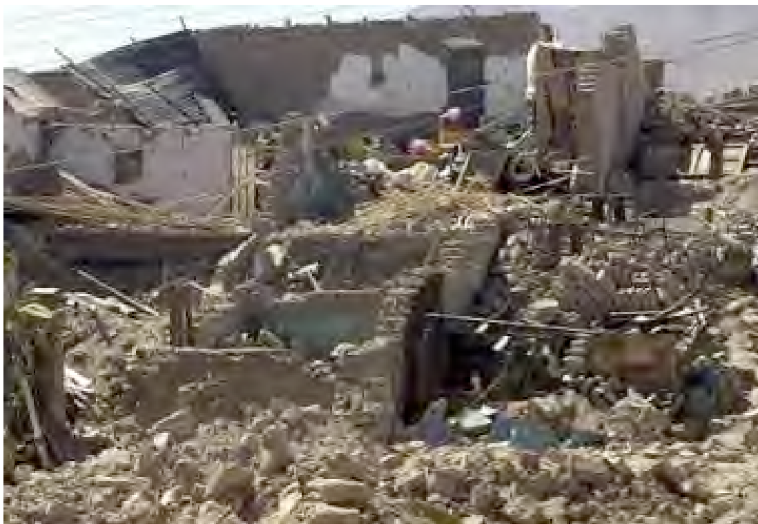
Figure 6. Extensive earthquake damage at Arequipa
