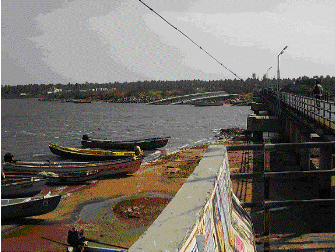
Photo 6. Damaged bridge is seen at rear center. Bridge on right is the new bridge.
