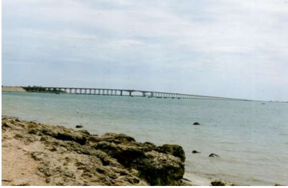
Mandapam South – Pamban bridge
