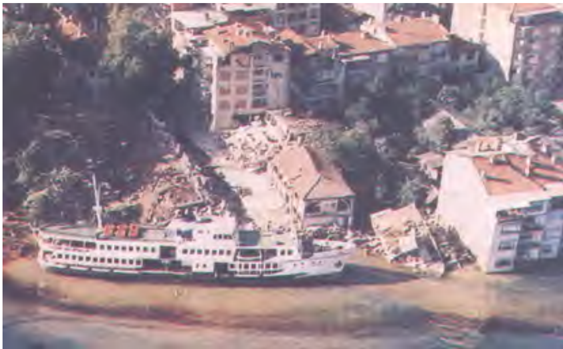
Fig. 10. Damage from the earthquake, tectonic subsidence, ground liquefaction and the tsunami. Ship in the foreground thrown onshore by tsunami wave action. Source: Kandilli Observatory and Research Institute (modified))
