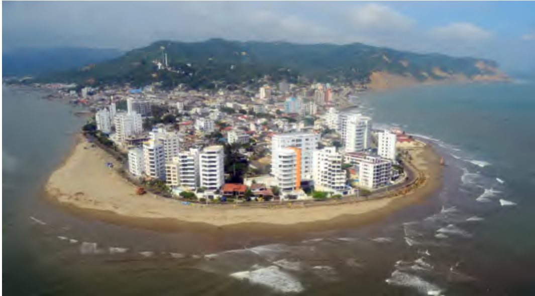
Fig. 5. Aerial panoramic view of Bahía de Caráquez, from north to south. Left side is the estuary of the Chone River, as well as part of the San Vicente – Bahía bridge and towards the right side is the Pacific Ocean.
