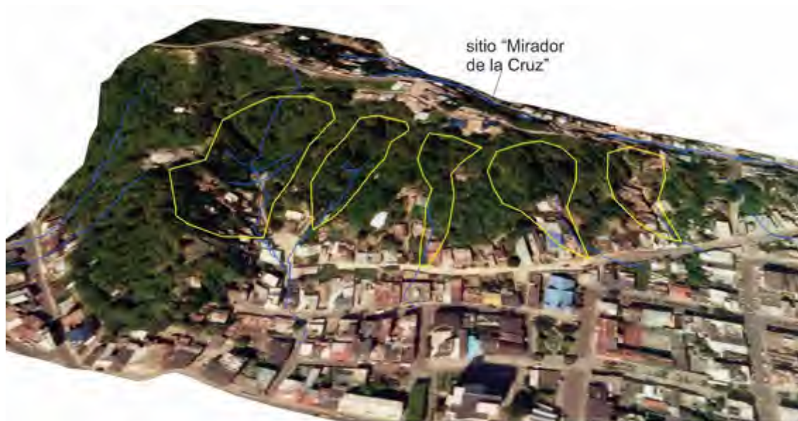
Fig. 6. Delineation of river sub-basins (yellow lines) characterized by intermittent streams, active only in winter seasons and “El Niño” phenomenon, and formation of deep furrows by incision of runoff waters on the slope, around the lower part of the “Mirador” de la Cruz site.
