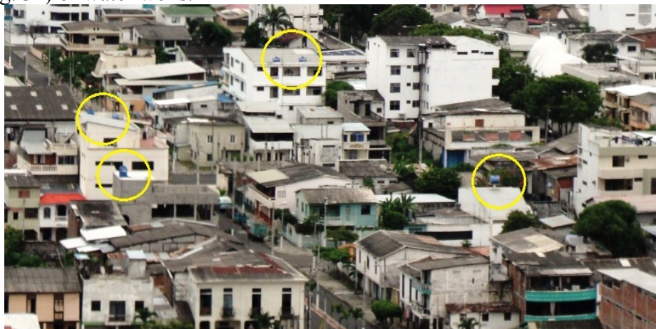
Figure 31: Cisterns in the medium vulnerability zone.
