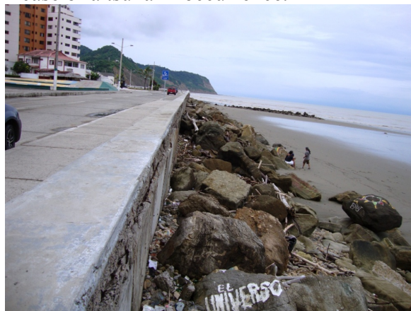
Figure 30: Protective wall in the western sector of the pier.
