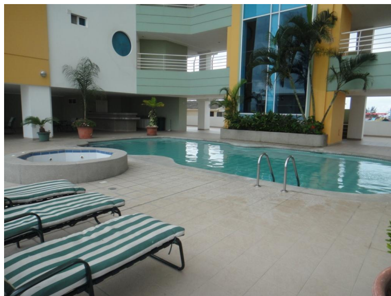
Figure 15: Communal services of the Riviera del Mar building (Salinas).
