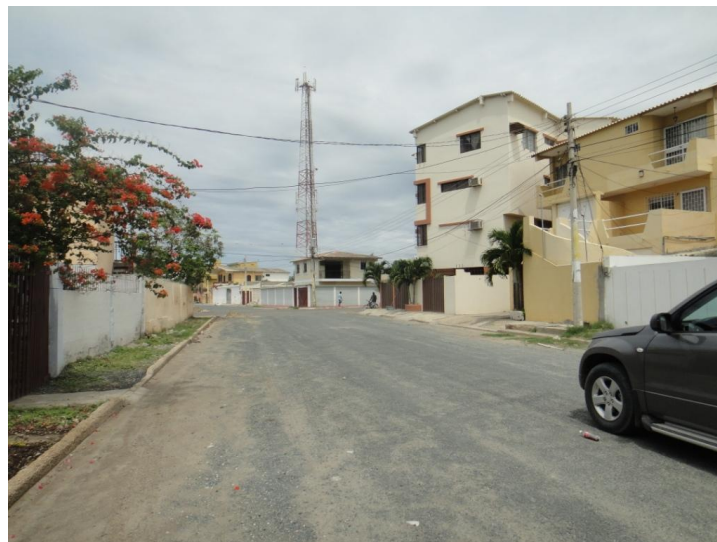
Figure 18: State of Salinas roads.
