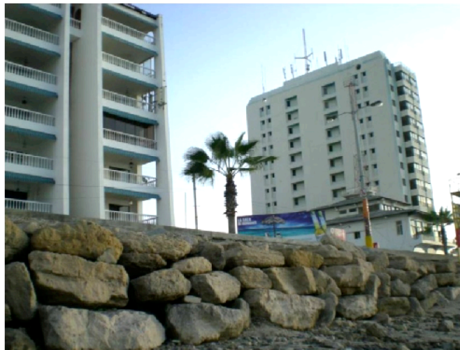
Figure 4: Cast rock-wall around the boardwalk of Salinas
