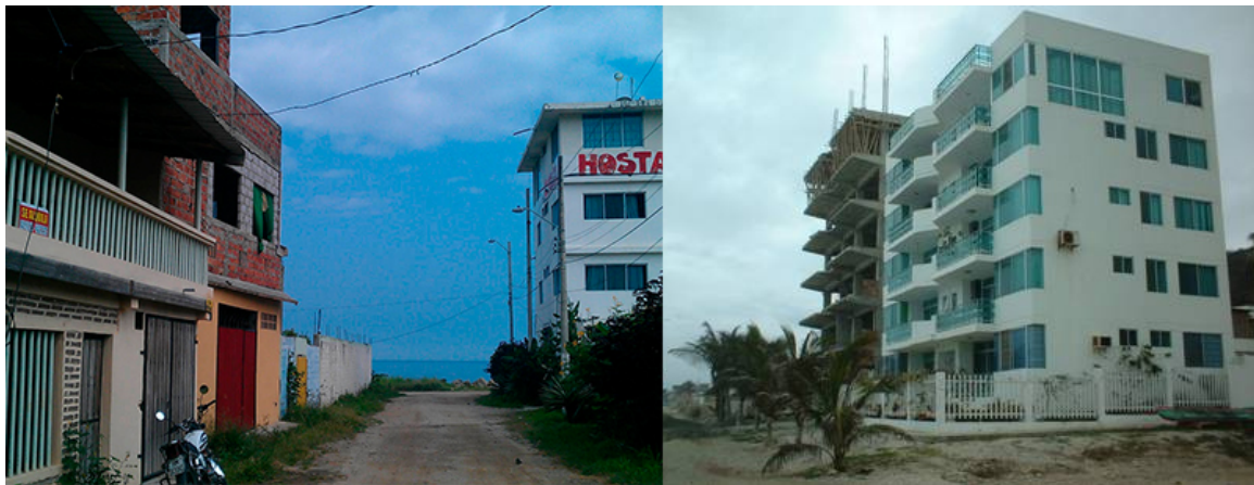
Fig. 7: Typical vulnerable buildings in the beach area of Crucita.
