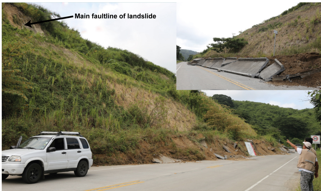
Fig. 15: Rotational slip in the road El Rosario – Canoa with evidence of escarpment at the slope and damages on the bicycle path and concrete road. Approximately 400 m 3 of material slipped (Chunga et al, 2016.). ESI Intensity = VIII and coordinates (UTM: 561.268mE 9.952.722mN).
