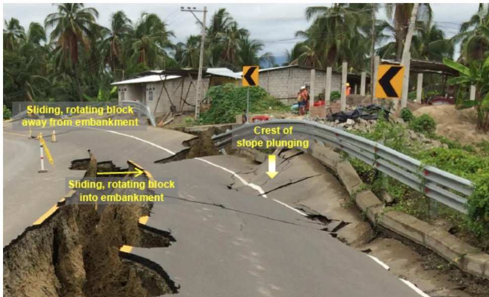
Fig. 29: Rio Chico: Settlement and rotation of block in foreground and circular global failure in background recorded by GEER-ATC (Nikolaou et al., 2016). (GPS: 0° 58' 36.6" S, 80° 25' 23.7" W).
