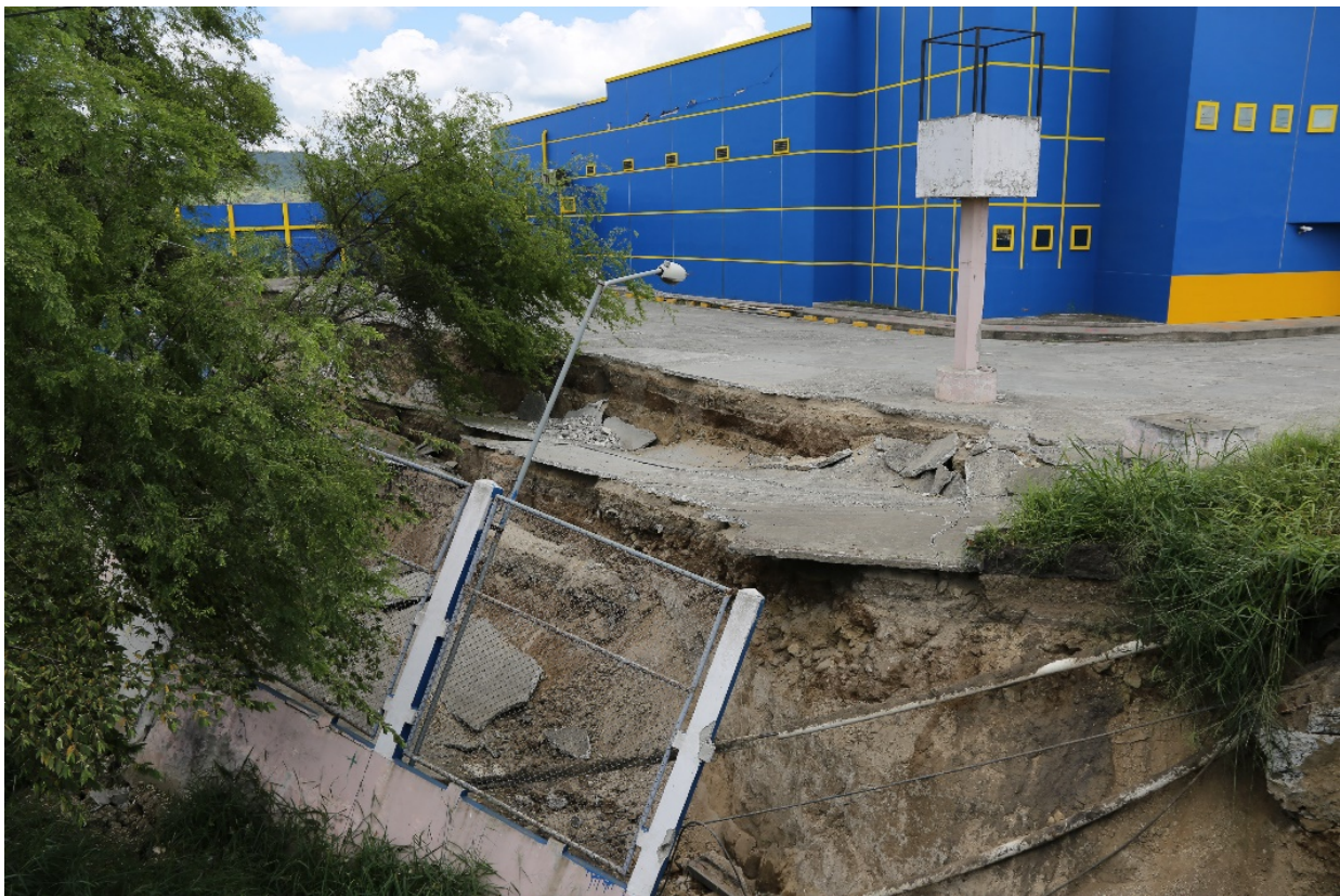
Fig. 27: Rotational and lateral ground deformations in the river margin, partial bridge collapse, easily eroded sandy material. Intensity ESI = VII. Bolvoni site, Portoviejo. 560261mE 9882769mN.
