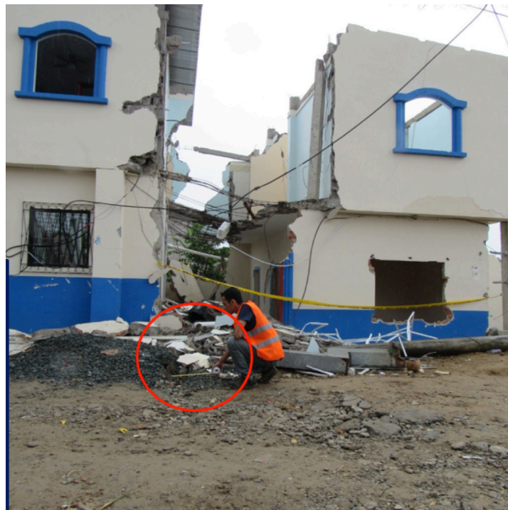
Fig. 20: In Chamanga cracks in natural terrain with openings of 15 to 25 cm and collapses of buildings. Intensity ESI = VIII. Coordinates UTM: 616034mE 10009804mN.
