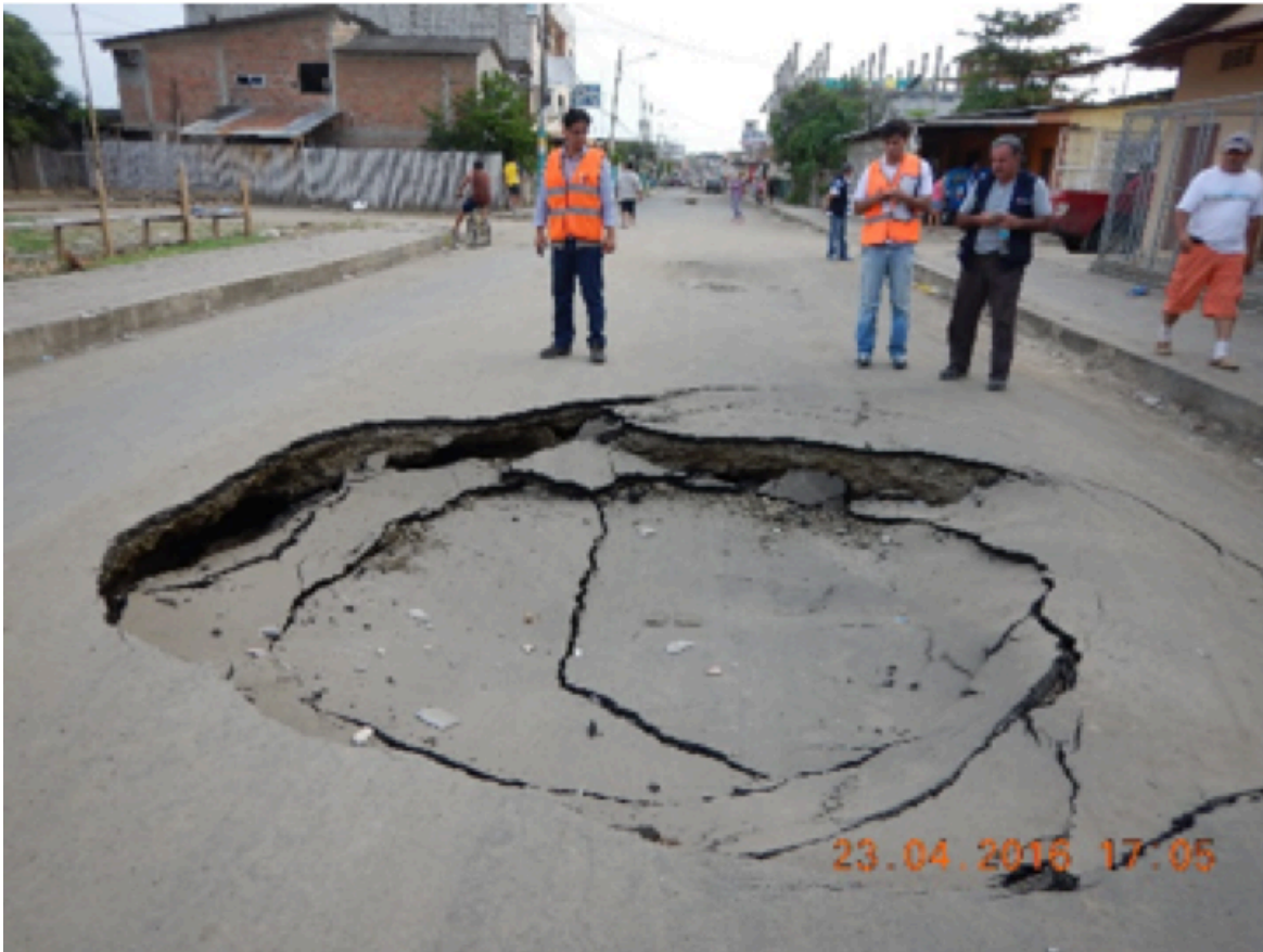
Fig. 24: Sinkhole at Tosagua village site with diameter of 2-3 m within floodplain and evidence of subsidence. Tosagua has been settling above an abandoned meander plain.
