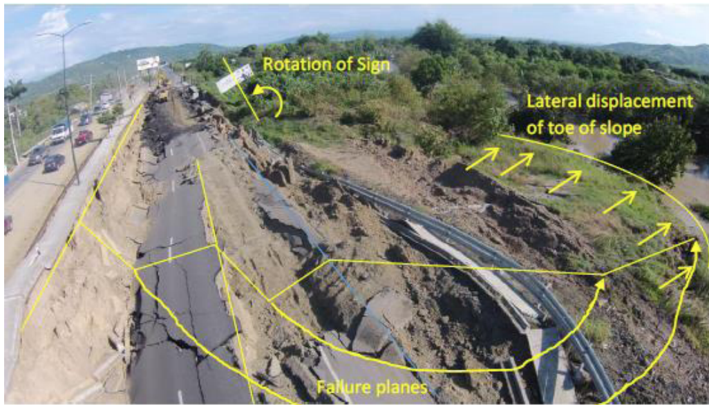
Fig. 19: Aerial view of embankment failure with assumed movement and failure modes marked with yellow at Mejia Bridge. Coord. UTM: 558.990mE 9.890.563mN. Intensity ESI = VIII. GEER-ATC report (Nikolaou et al., 2016).
