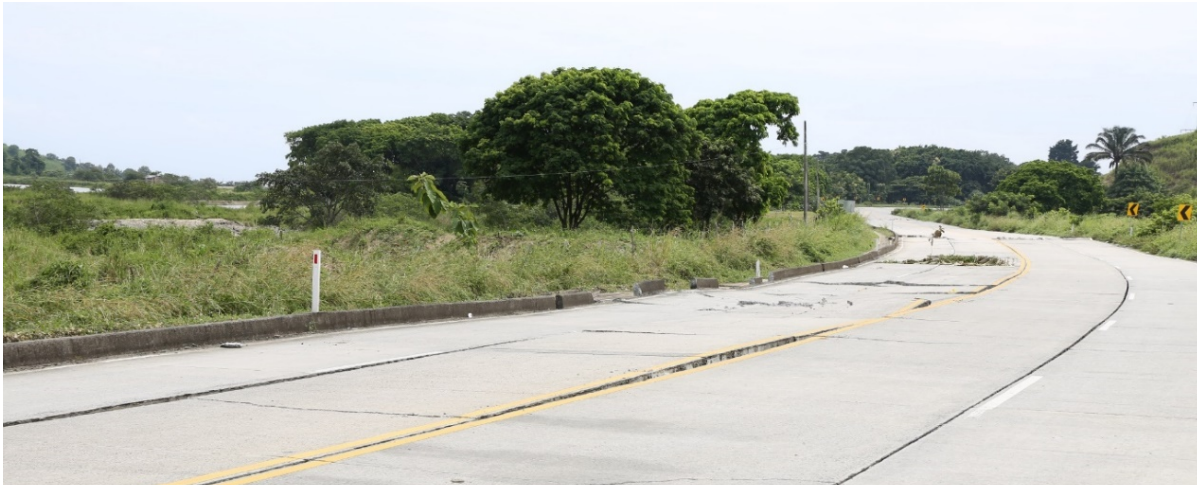
Fig. 9: Deformations along concrete-made road between Pedernales and Coaque, with diagonal and transverse fractures 10 to 14 cm wide. geomorphological floodplain features. ESI Intensity of IX and coordinates (UTM: 602.858mE 10.003.638mN).
