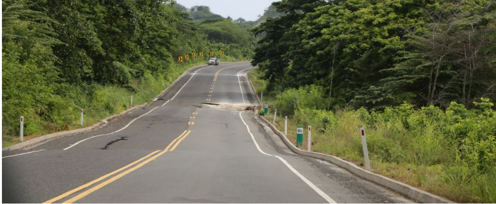
Fig. 11: Deformation in Jama paved road, with transversal fractures 20 to 30 cm wide and longitudinal fractures of 12 to 15 cm. Cracks observed in the free field soils reached 1 m. ESI Intensity of IX and coordinates (584.676mE 9.982.122mE).
