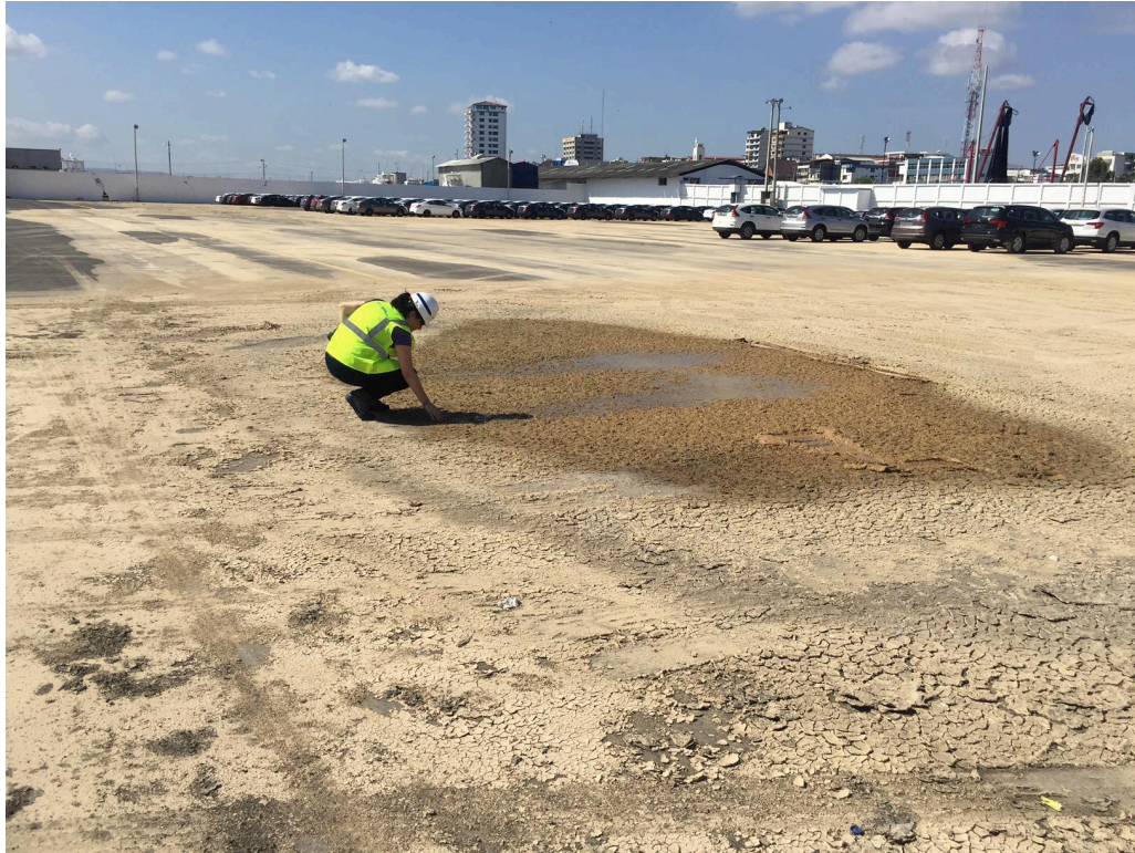
Fig. 30: Concentrated sand blow in the center of pavement in the Manta Port parking area (GPS: 0°56'27.6"S, 80°43'29.4"W). (Nikolaou et al., 2016)
