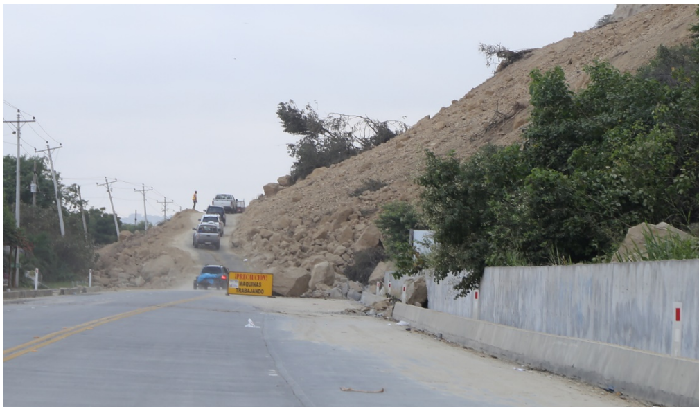
Fig. 17: Massive rockfall, which covered and destroyed completely the paved road with some 10,000 m 3 at Boca de Briceño. Intensity ESI = VIII, coordinates (561.647mE 9.944.416mN).
