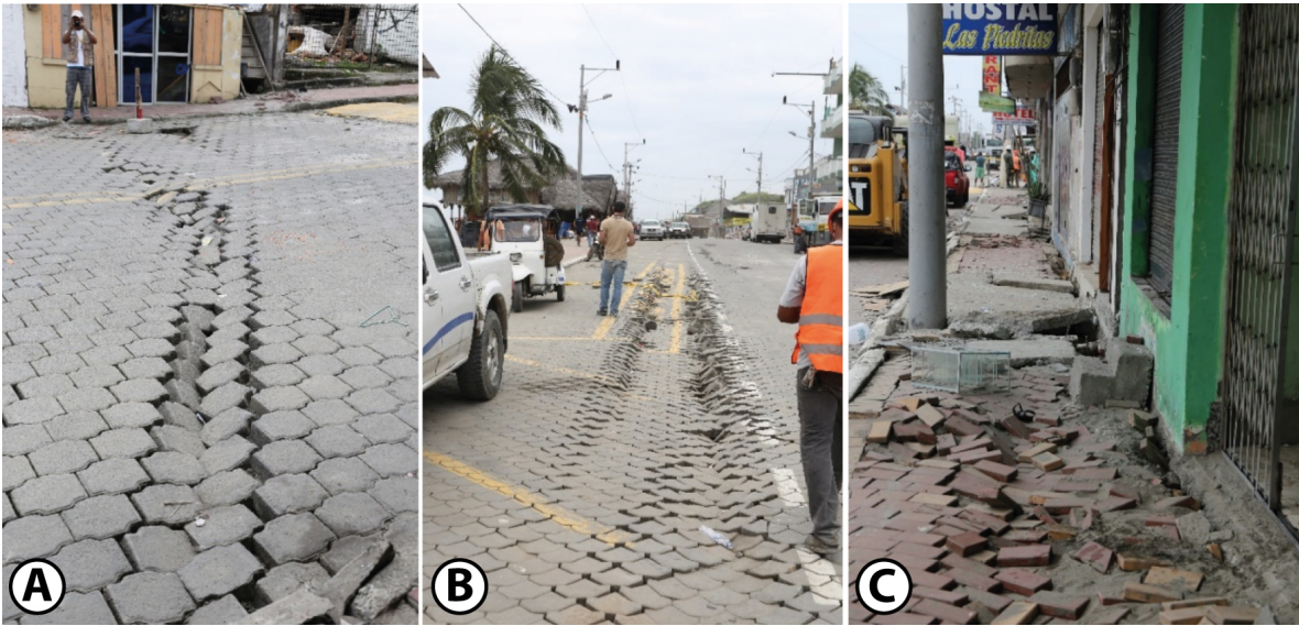
Fig. 10: Wavy deformations on the beach boardwalk and streets of Pedernales, with re-arrangements of cobblestones in folds. ESI Intensity of IX to X and coordinates (UTM: 604.756mE 10.007.656mN).
