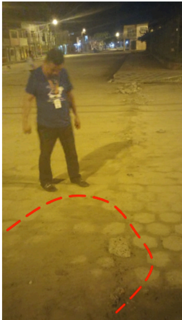
Fig. 21: Liquefaction evidence in the central park of Muisne Island. Intensity ESI = VIII and coordinates (UTM: 609170mE 10067485mN).
