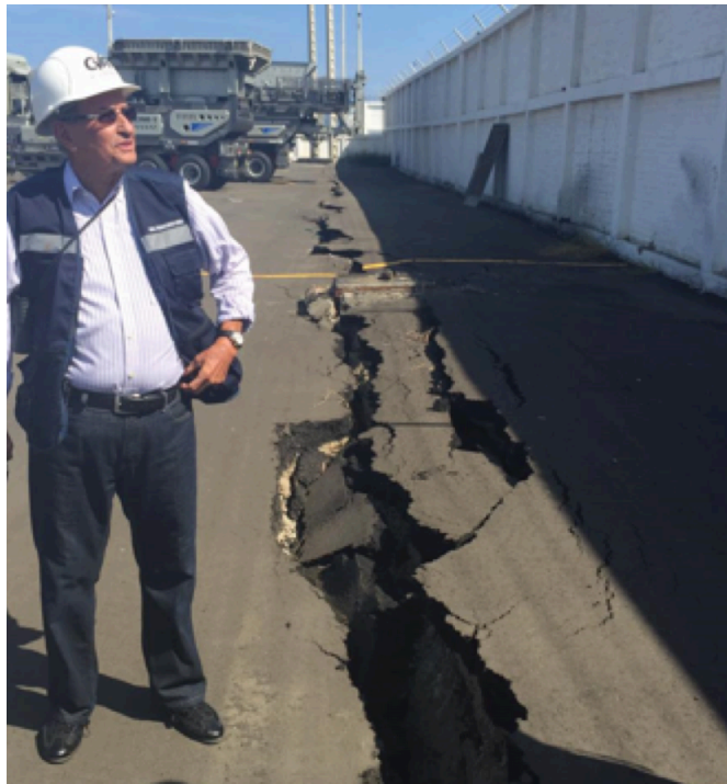
Fig. 26: Longitudinal fractures in middle of a paved road in Manta, with openings of 2 to 5 cm, lateral spreading. Coord. UTM: 531735mE 9894912mN.
