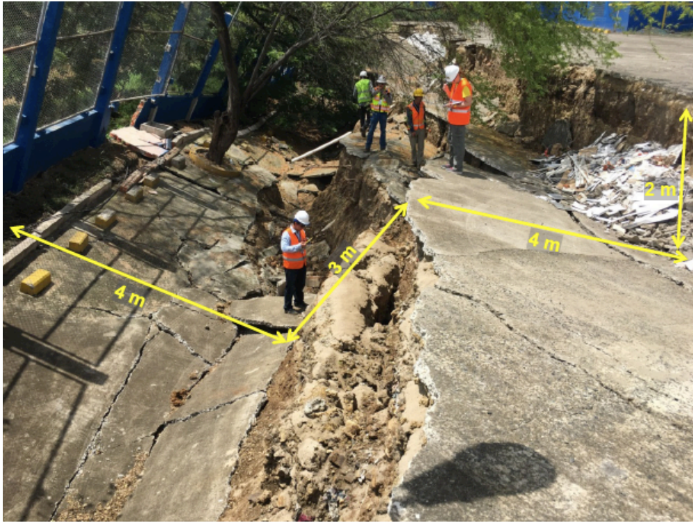
Fig. 28: Wall at Portoviejo Velboni site recorded by GEER-ATC (Nikolaou et al., 2016): Slope failure showing two primary slip surfaces and wall rotating, following the slope movement (GPS: 1°3'37.8"S, 80°27'29.3"W).
