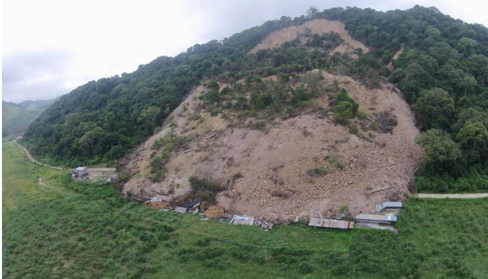
Fig. 16: Aerial photo of landslide on San Vicente-Canoa local road by GEER (Nikolaou et al., 2016). (GPS: 0°33' 5"S, 80°25'42"W UTM coordinates 9939051.9N, 563610.3E)
