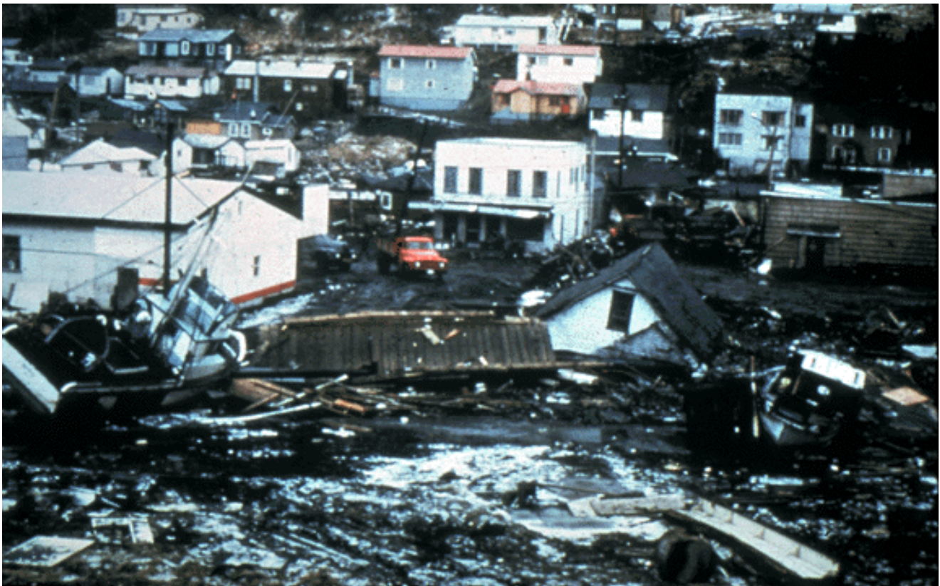
Fig. 5 Photo of the 1964 tsunami damage at Port Alberni, British Columbia, Canada
