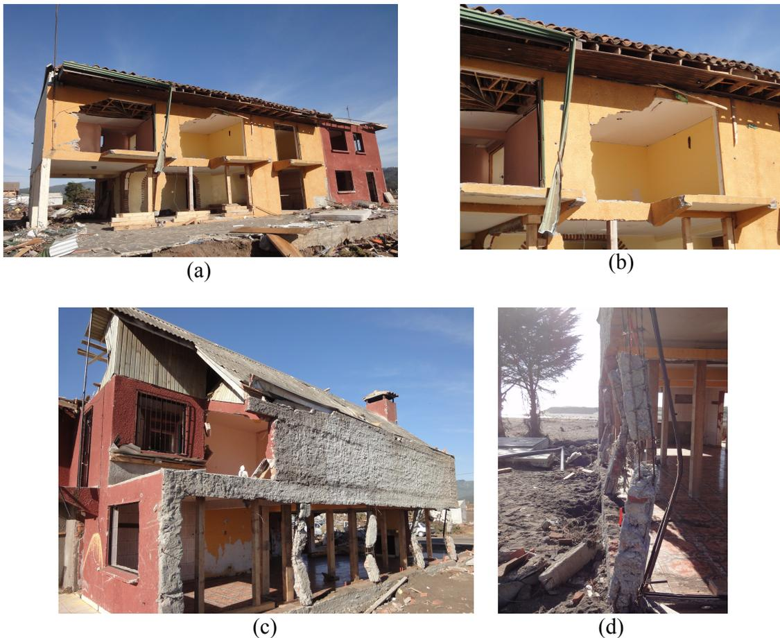
Figure 2. Effects of 2010 Chile tsunami on residential structures in Pelluhue (Palermo et al., 2013): a) global damage to two storey-structure; b) punching failure of second storey masonry infill walls; c) damage to masonry infill walls and loss of load bearing elements at first storey level; and d) destruction of lower level columns.
