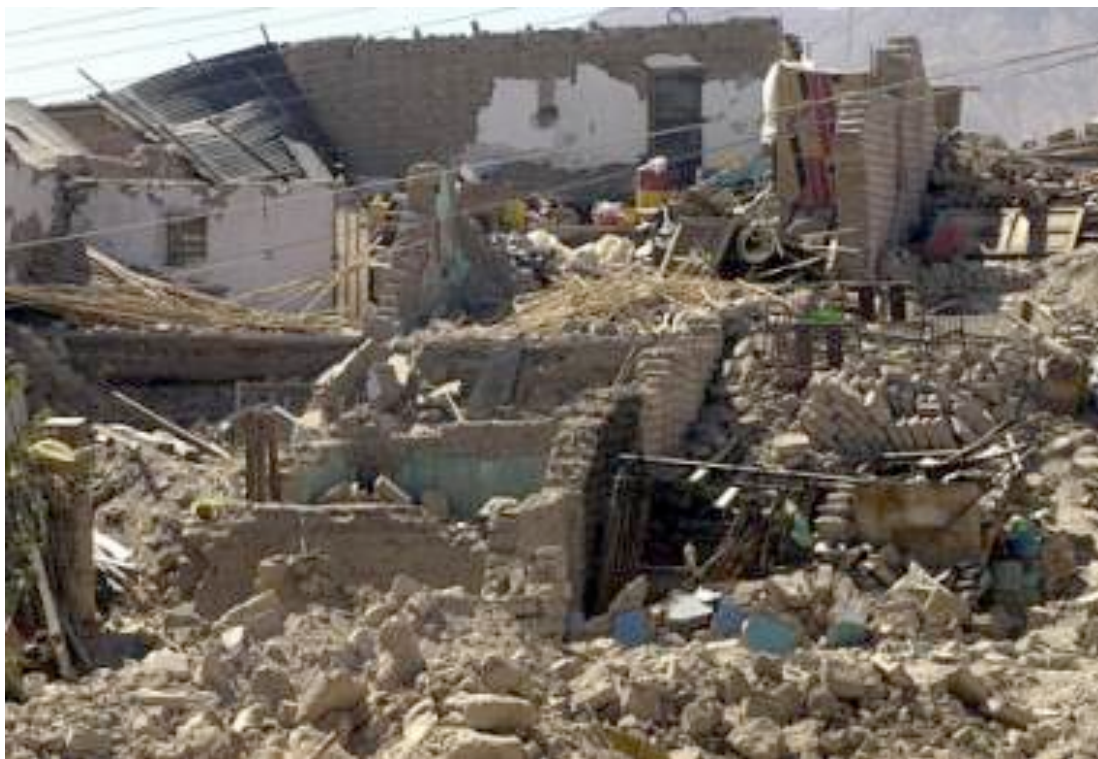
Figure 6. Extensive earthquake damage at Arequipa
