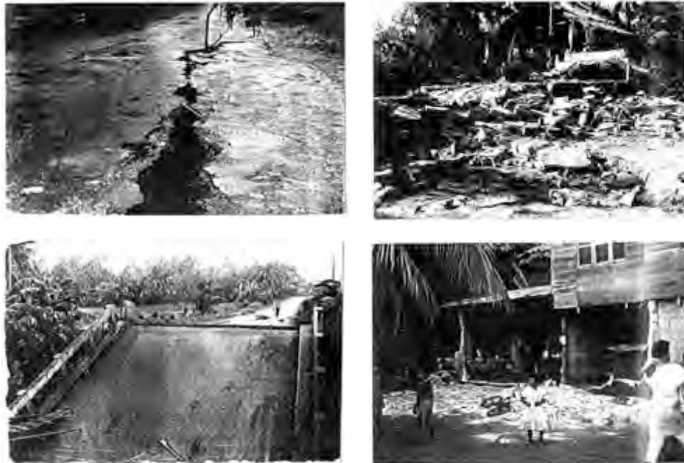
Figure 4a: Photos adapted from Umbal et al. (1990) showing the damages at Guindulman (A), fault rupture near Anas (B), the collapsed bridge at Alijauan bridge at Jagna (C) and collapsed house in Candabang, Anda (D).
