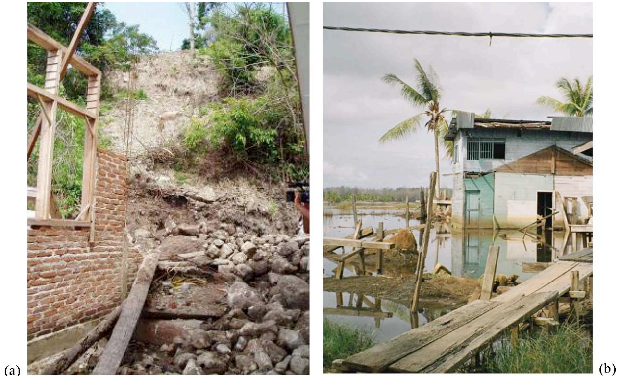
Figure 2 Examples of housing a risk due to non-tsunami hazards (a) landslides due to rainfall (b) inundation by the sea
