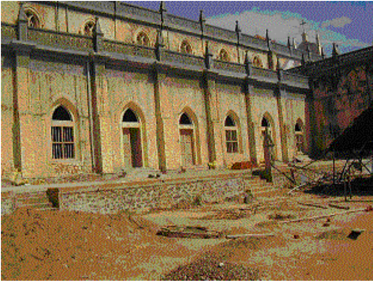
Photo 4. The repairs on first floor indicate damage during tsunami and the level of Tsunami height.
