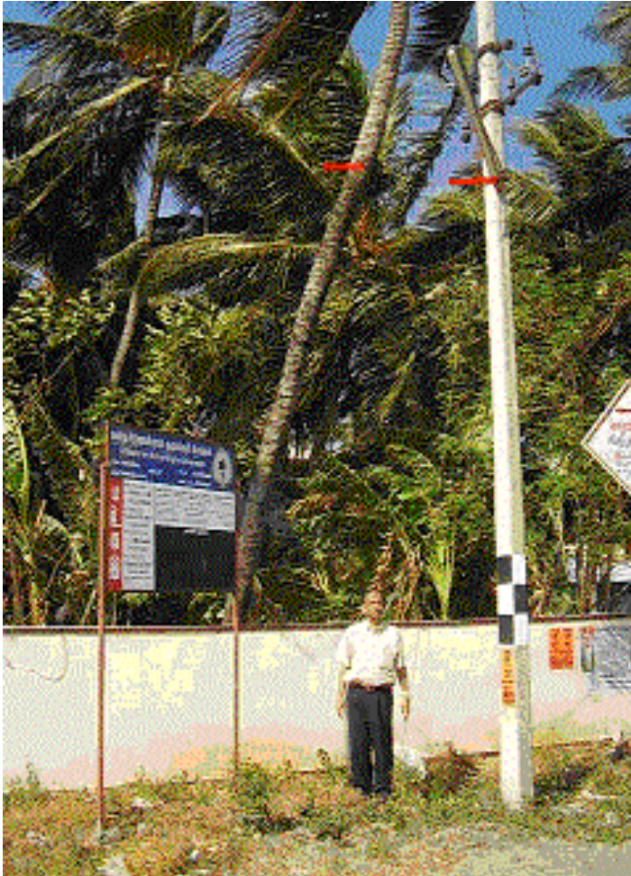
Photo 1. Shows the tsunami mark on the coconut tree and metallic part on the electric lamppost, which have been corroded.
